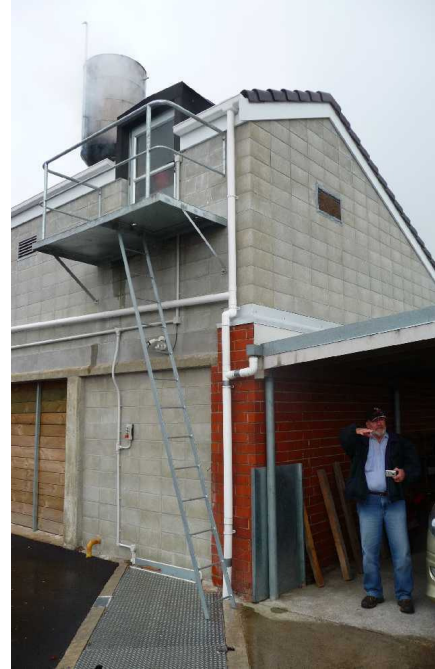
Little Sisters of the Poor storage for 300kW Binder boiler
